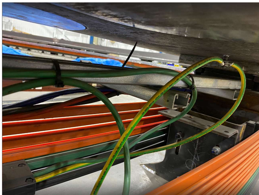
Typical Under-Track Brackets and Grounding Cables to be Salvaged
