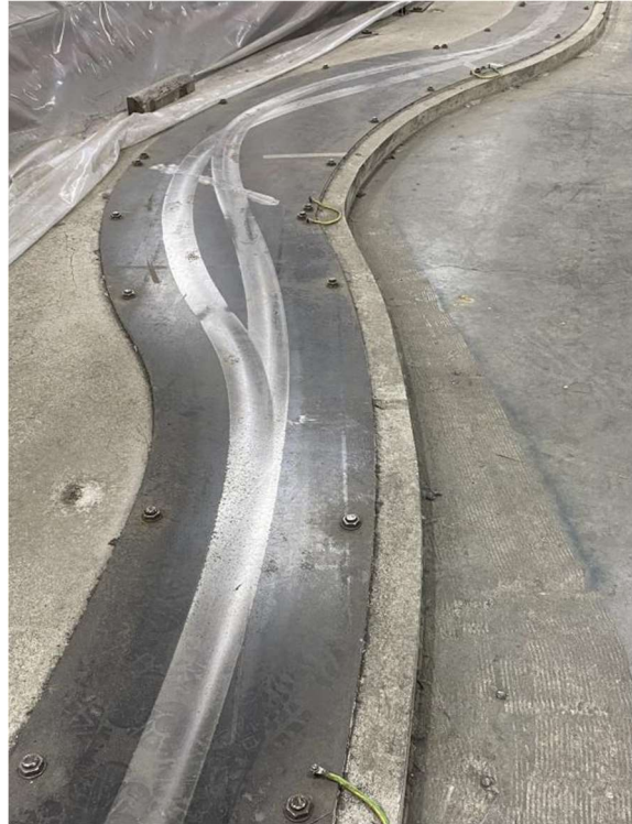
Typical Under-Track Brackets and Grounding Cables to be Salvaged
